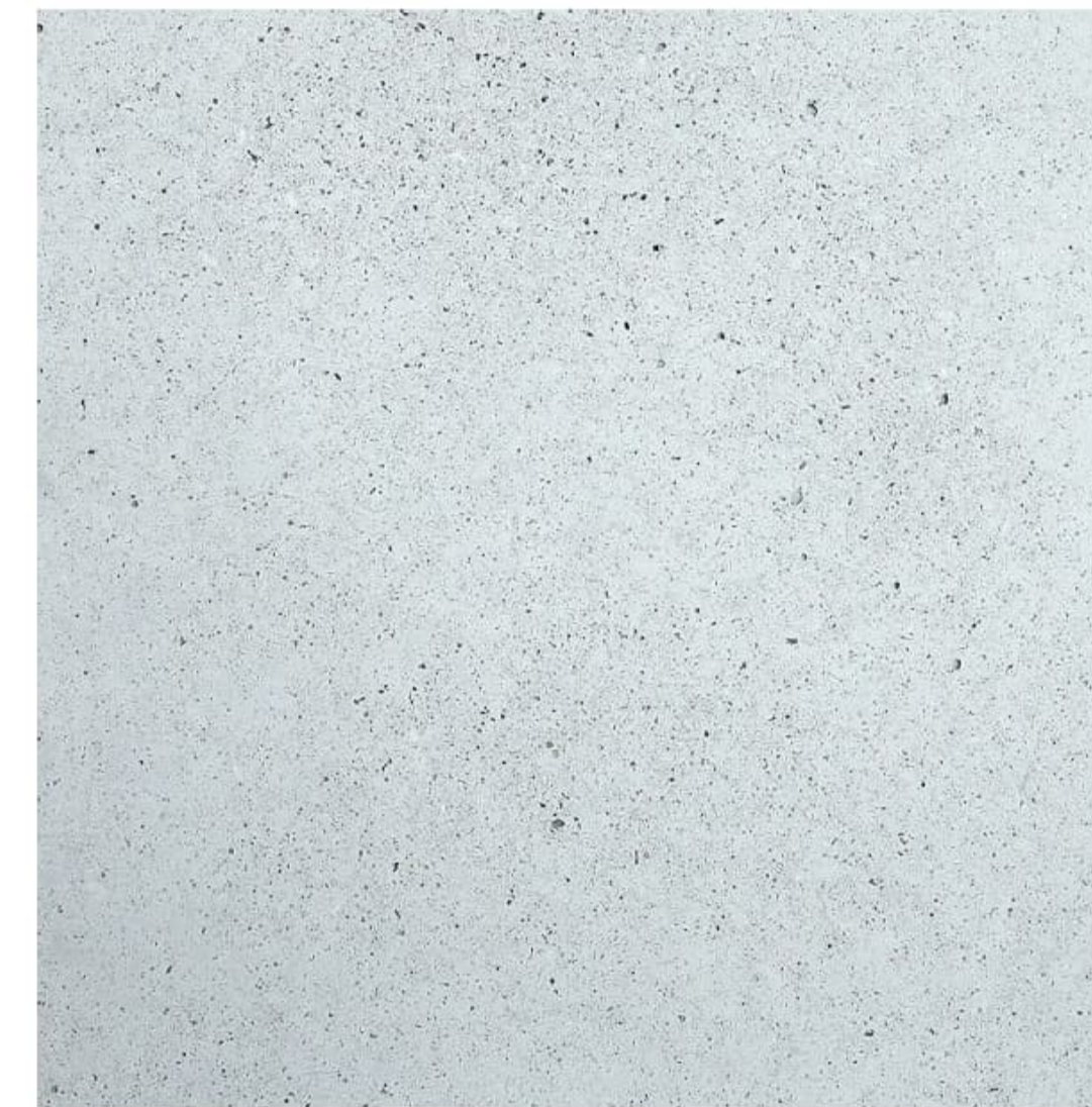
Natural Finish Hardstand Concrete
