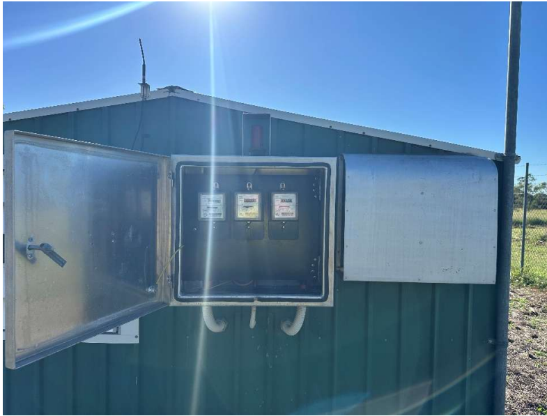
Figure 2: Ergon Metering Panel & Comms Antenna to be Retained
