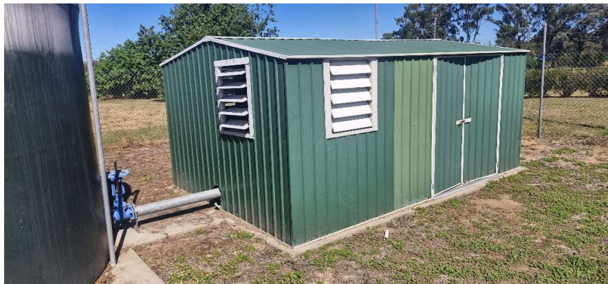
Figure 1: Existing Pump Shed
