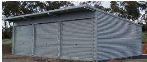
Skillion roof design with roller doors opening to playing fields
