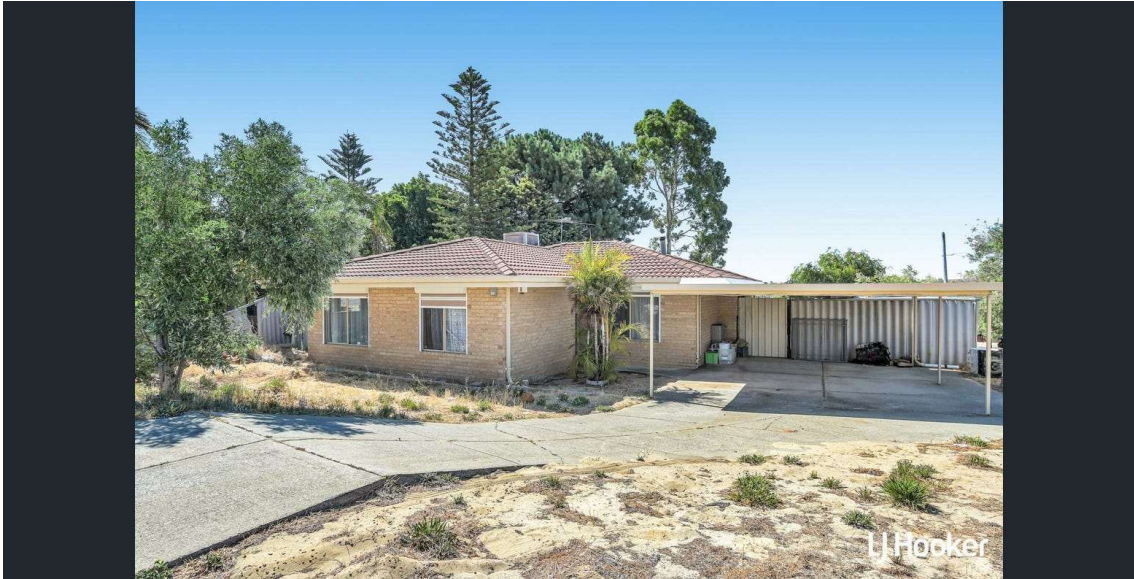
Figure 2 Existing carport front view
